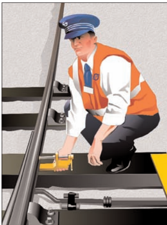
Step 5 shows an image of a clip under the other rail
